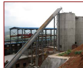
New Mill under Construction
