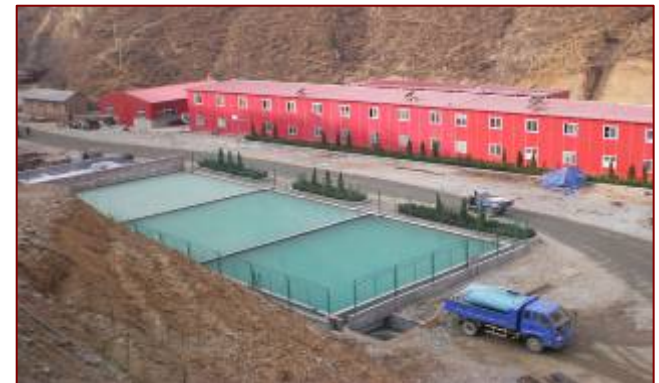
Mine water from the SGX mine flows into a three-stage, centralized settling pond. Discharged water meets Class II water standards.
