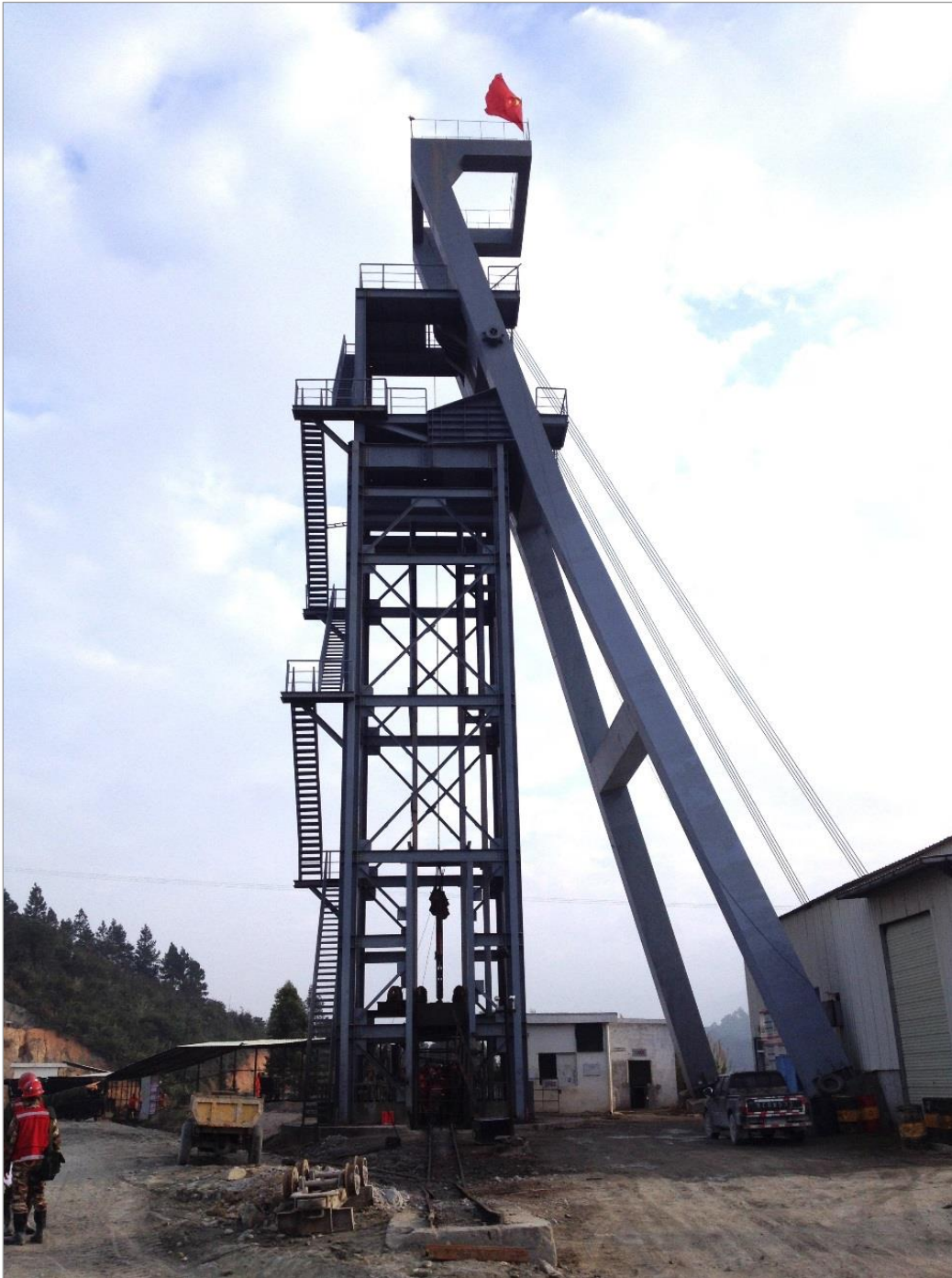
Figure 16.10 Main Shaft headframe
